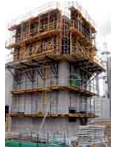
CM-220 brackets with ORMA vertical formwork
