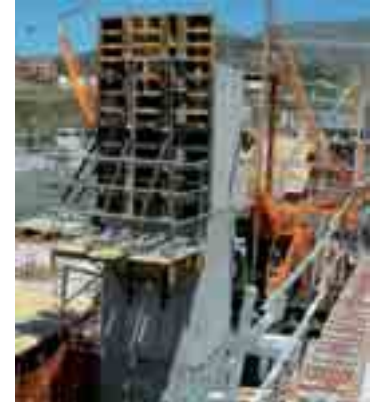
BF-170 brackets with ORMA vertical formwork
